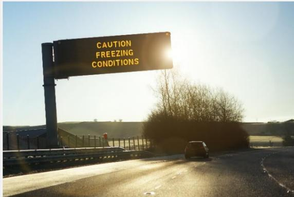
Figure 4-16: Cantilever VMS sign
