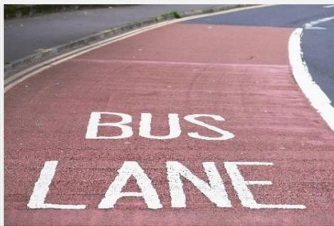
Figure 4-12: Bus Lane with coloured surface
